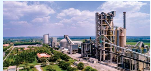
Binh Phuoc Cement Plant
